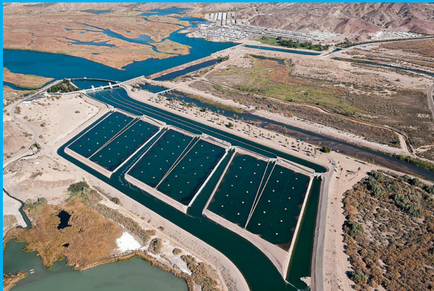
All American Canal Diversion Dam (USBR)
